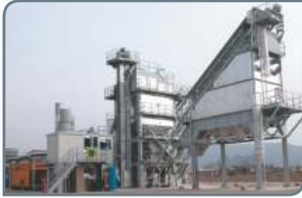
ASPHALT BATCH MIX PLANT
